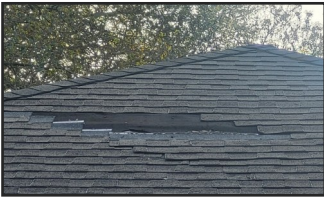
Forsamlingshus roof damage caused by March storm. Full roof replacement on both buildings followed soon thereafter.
