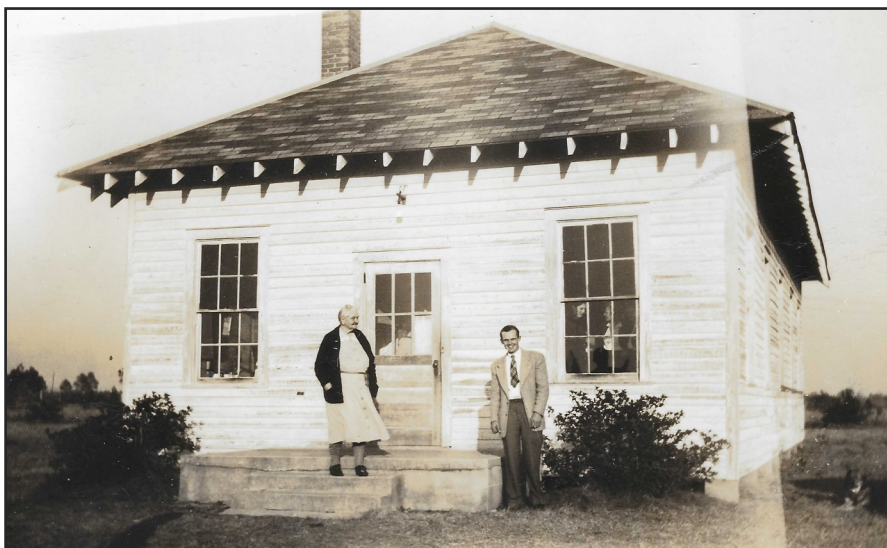
The forsamlingshus circa 1942. Pictured are Sine Nygaard visiting from Danevang and Granly resident Paul Pedersen. The photo shows the original brick chimney that was connected to a pot bellied wood stove used for heating the building. The landscape then was very different with open farmland and very few trees. In the Dannevirke article Pastor Frost wrote that the building “can be seen from almost every home there”.
