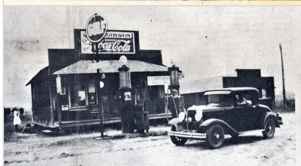
Pictured above with his family, Hurley resident J.B. Gibson was instrumental in helping early colonists get started. He owned the general store pictured above and allowed new arrivals to stay in the building next door until their new homes were completed. Photos provided by descendants J.B. Gibson.
